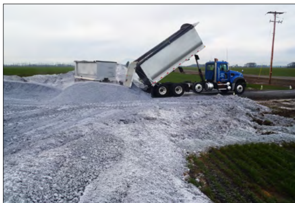
Figure 16.—Delivery and piling of by-product lime.
